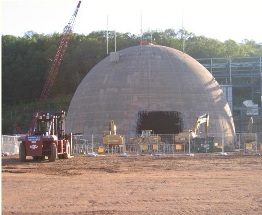
Figure: Demolition of Containment Building
