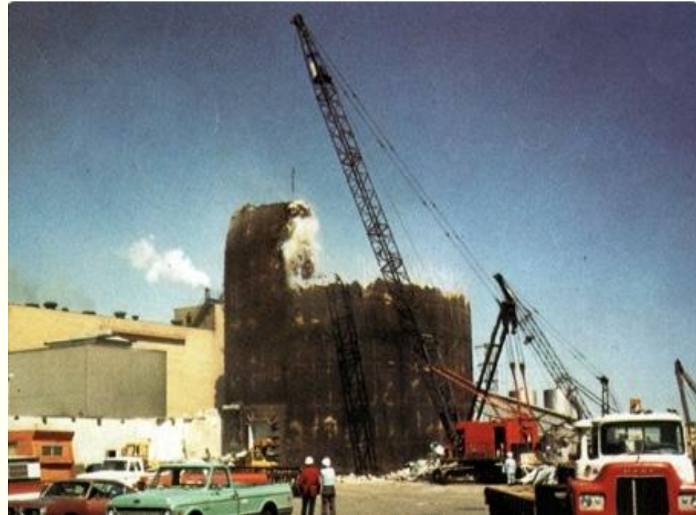
Figure: Demolition of Containment Building
